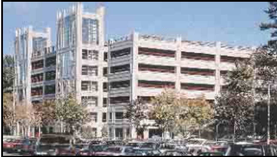
Figura 2.10 – Boston College Parking Structure, Chestnut Hill, Massachusetts – USA.
