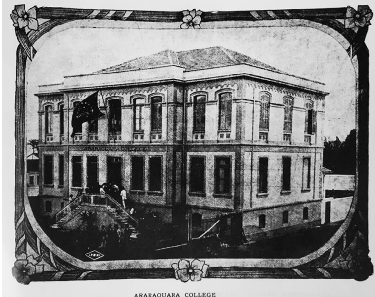
Figura 67 – Vista externa do Araraquara College.
