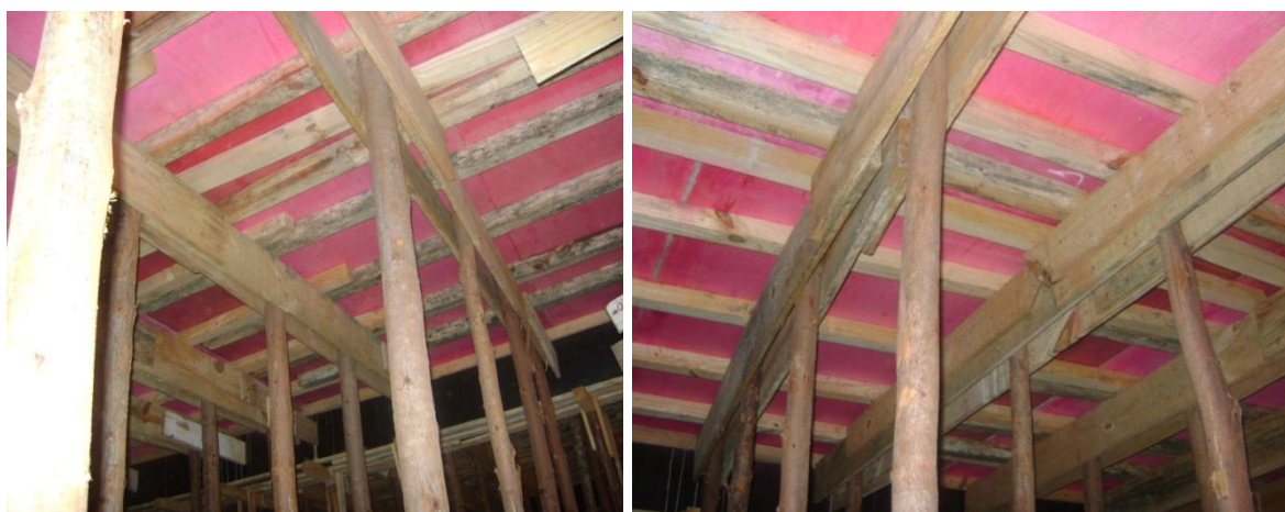
Figura 49 – Longarinas apoiando as transversinas
