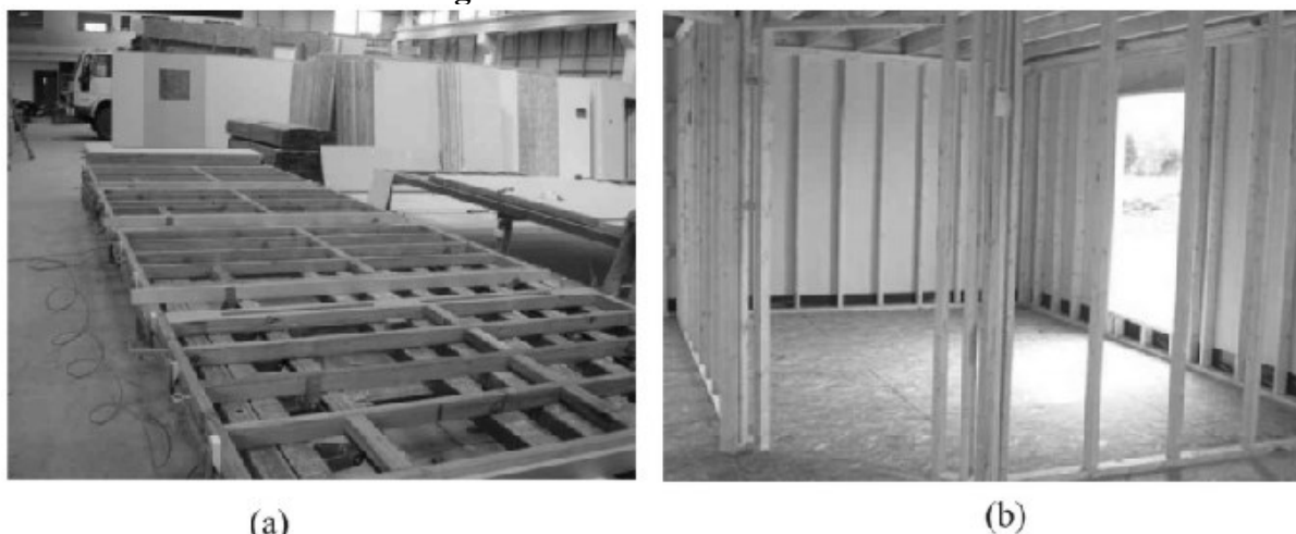
Figura 3 – Painéis Wood Frame
