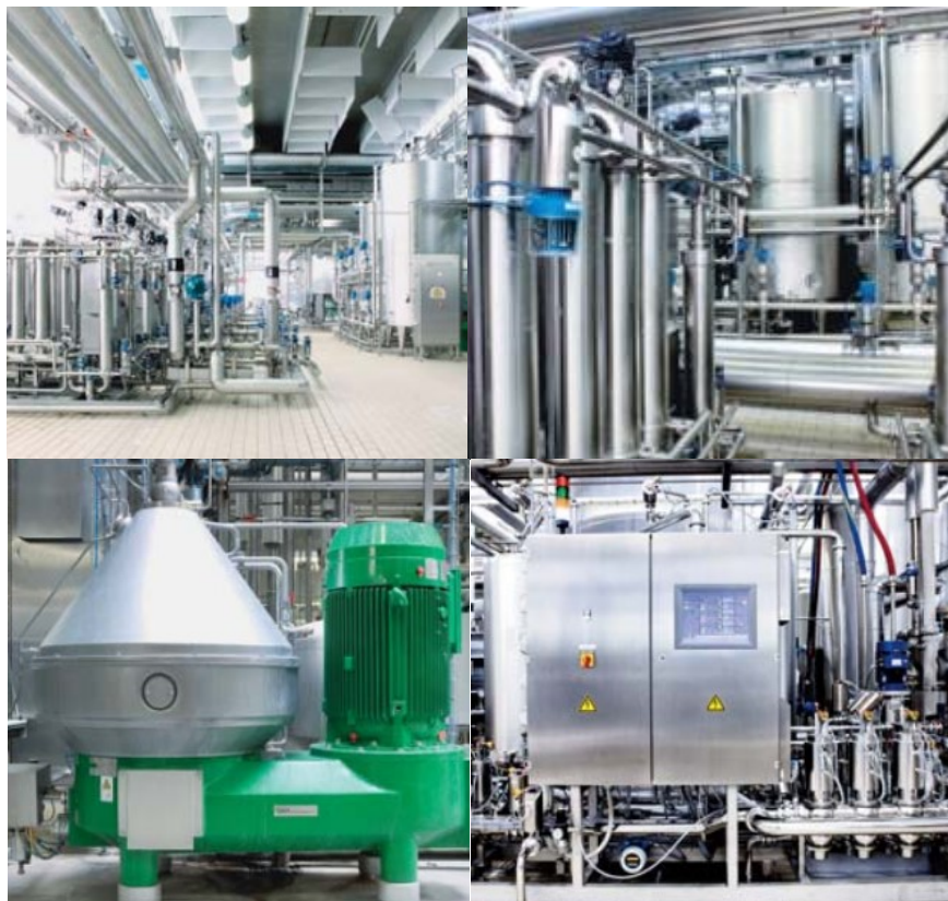
Figura 3.7 – Sistema de membranas de fibra oca de PES instalado. Fonte: < www.shop.pall.com/us/en/food-beverage/beer-corporate-/clarification/profi-membrane-system-for-de-free-clarification-of-beer-zidgri78lkm >.
