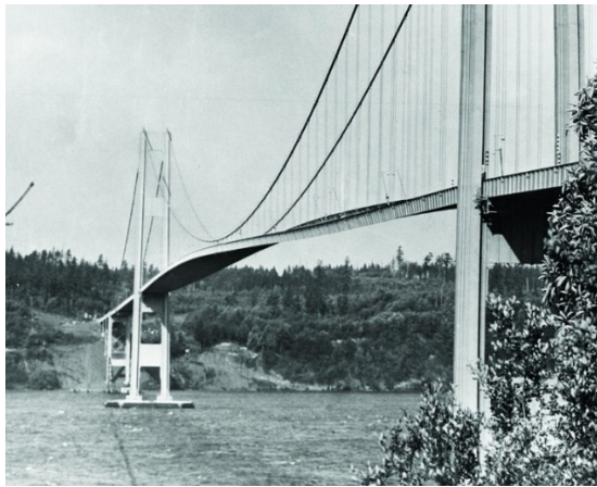
(a) Tacoma Narrows Bridge.
