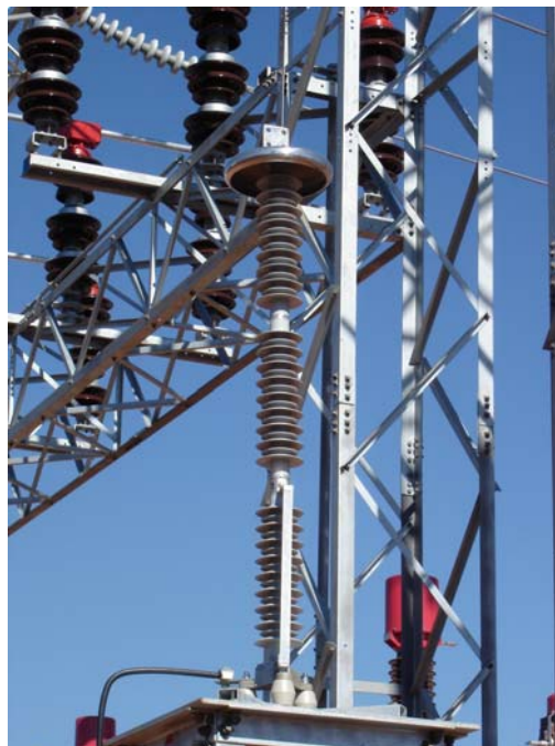
Figura 2.18 – Para-raios 138/88 kV
