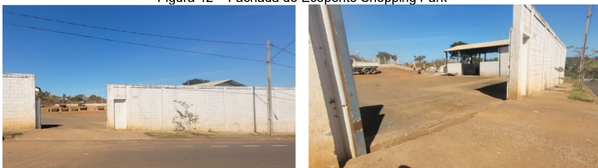
Figura 42 – Fachada do Ecoponto Shopping Park
