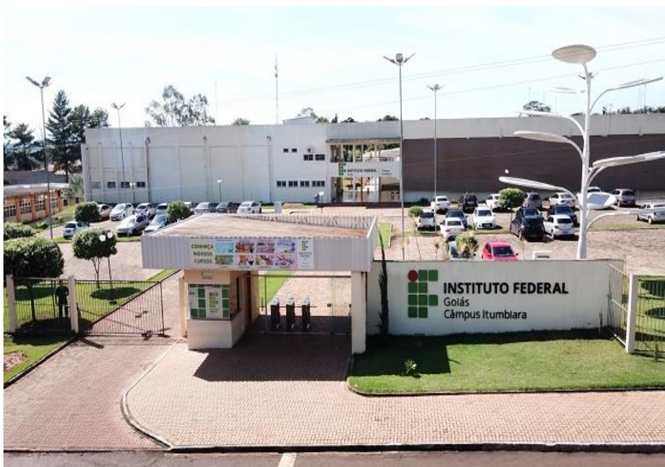
Figura 2 – Fachada do IFG/Campus Itumbiara
