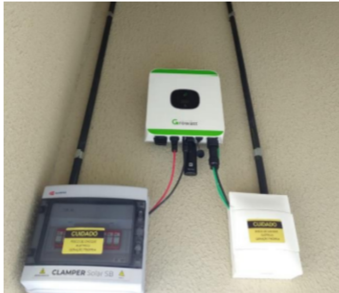
Figura 34 – Inversor instalado
