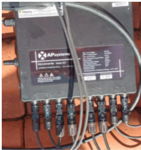
Figura 36 – Microinversor instalado
