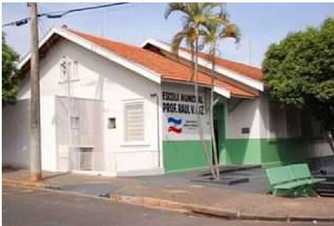
Figura 02 – Escola Municipal Prof. Raul Vieira Luz - Fonte: https://www.google.com/url?sa=i&url=https%3A%2F%2Fwww.facebook.com%2FRaulVieiraLuz%2F&psig=AOvVaw2y-4YHrK29bU6bB7uwFd24&ust=1634322069835000&source=images&cd=vfe&ved=0CAkQjRxqFwoTCLilmKjCyyMCFQAAAAAdAAAAABAD Acesso em outubro de 2021
