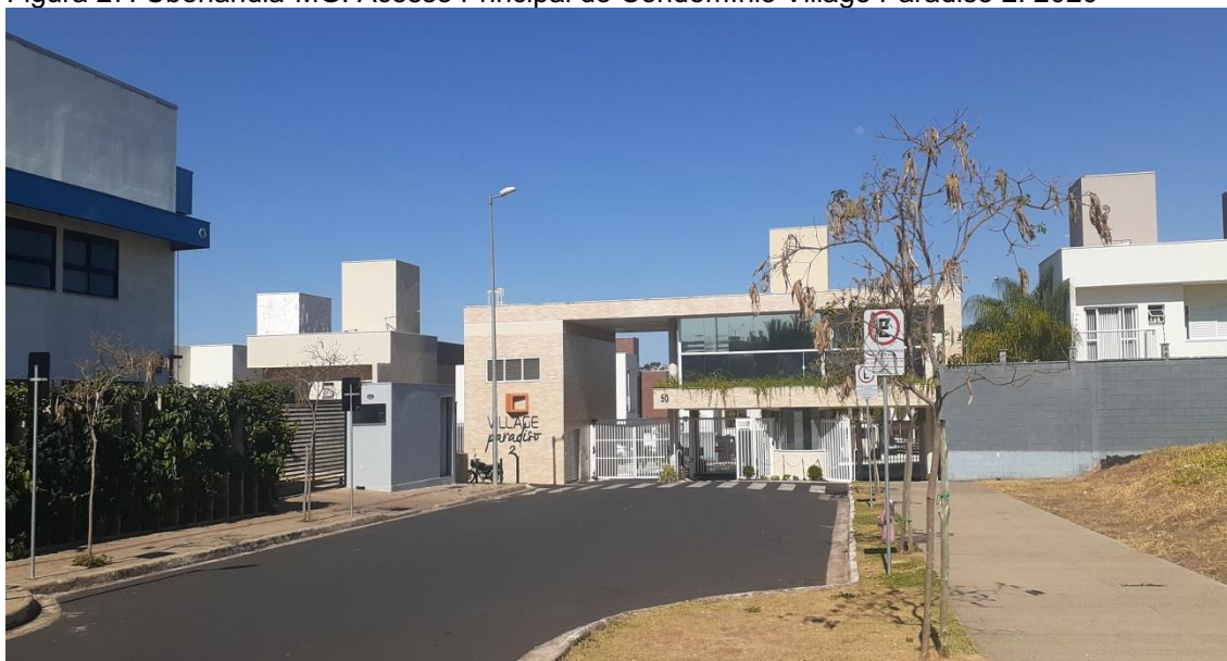
Figura 27: Uberlândia-MG: Acesso Principal do Condomínio Village Paradiso 2. 2020
