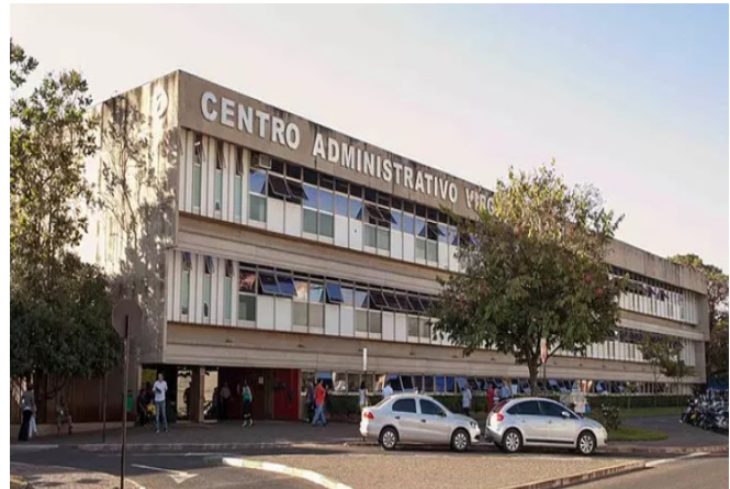
Figura 11: Centro Administrativo Municipal (2019)
