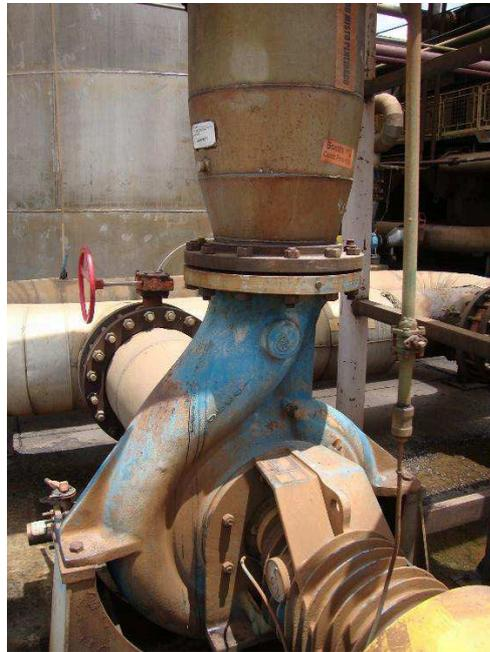
Figura 3.5 - Bomba centrífuga radial EQUIPE EQP
